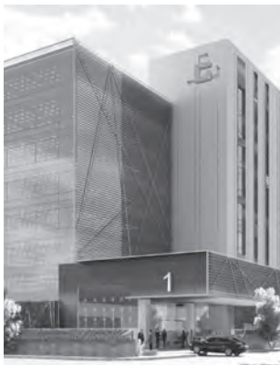
Gigaplex IT Building
