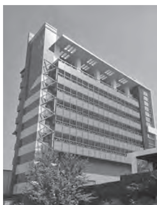
Airtel Mobile Switching Centre
